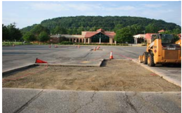
Middle School Asphalt
